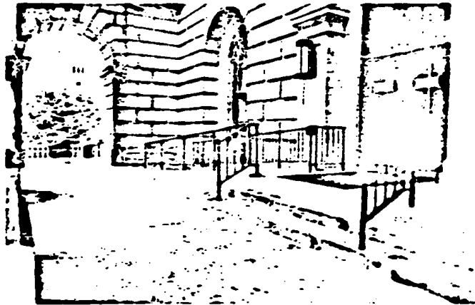
A good example of a curved approach and level area in front of entrance doors.
