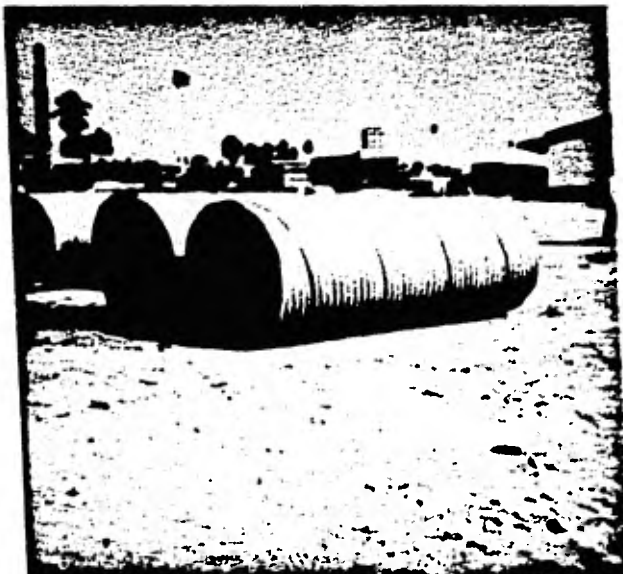
Fig. III.7 Cimbra metálica (Spiroform).
