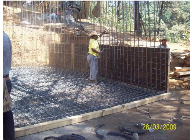
Encofrado de tanque mayor
