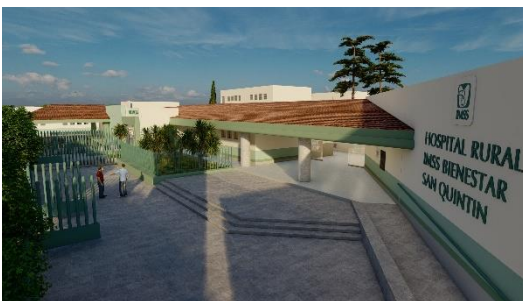
Vista general del Hospital
