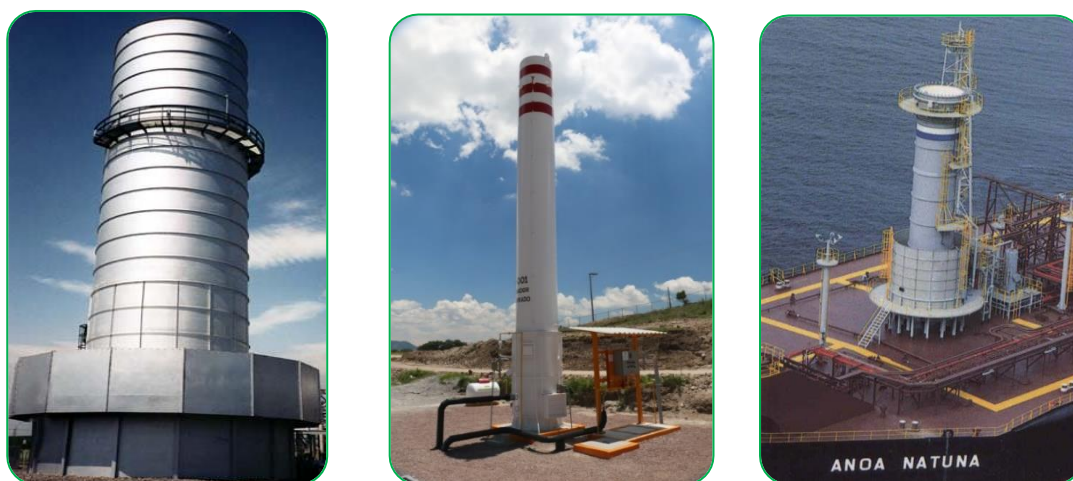
Fig. 2. Onshore & Offshore applications of Enclosed Ground Flares (EGFs)
