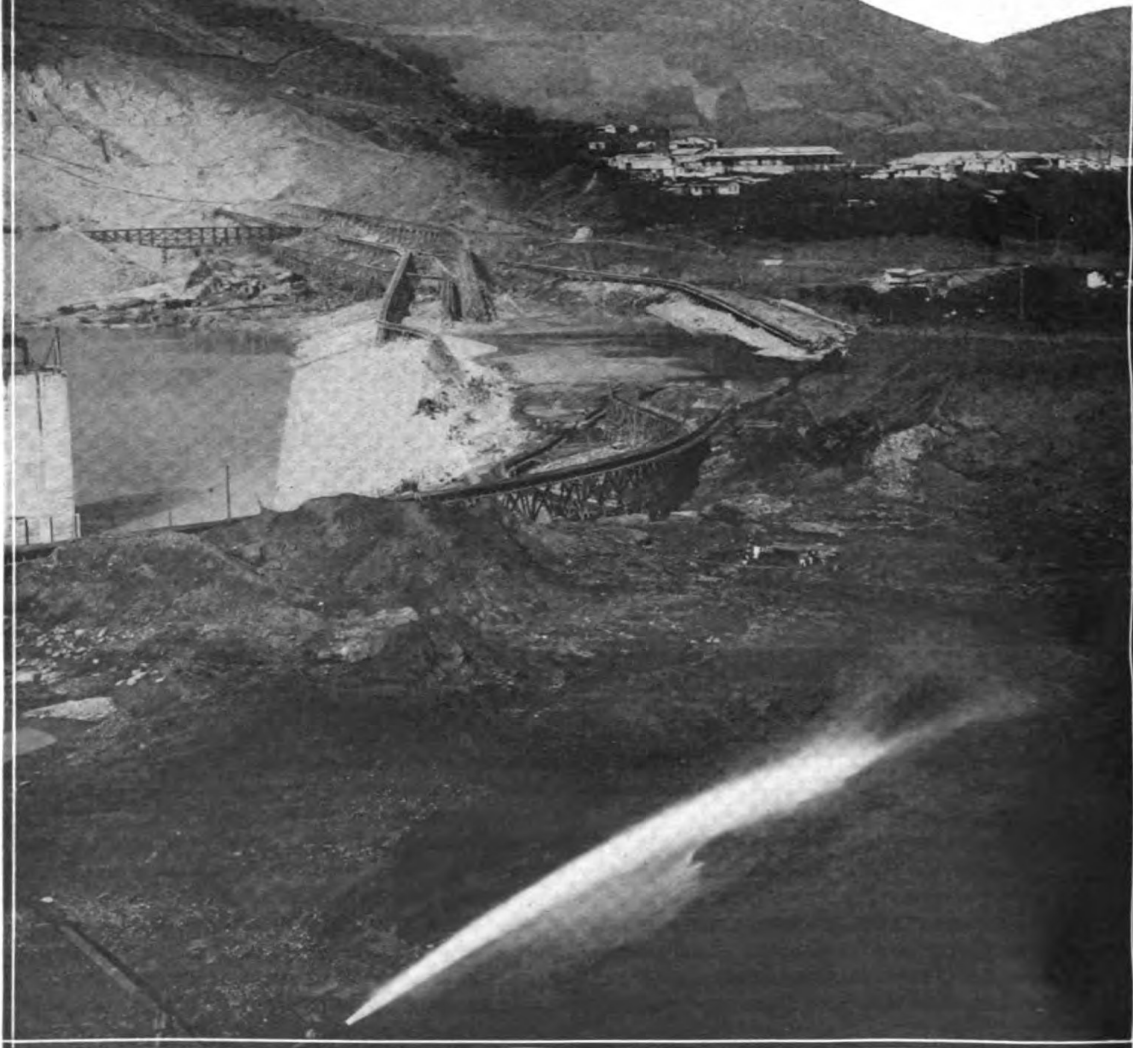
THE NECAXA DAM UNDER CONSTRUCTION.
