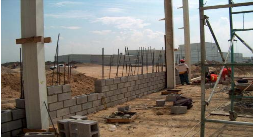
FIG.II.5.4 MUROS DE BLOCK
