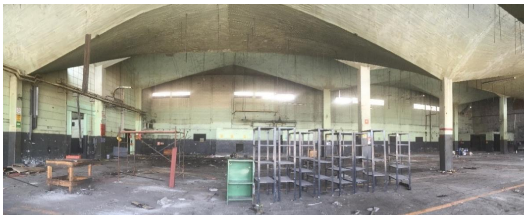
Losas bodega principal
