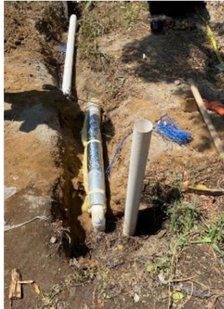
Figure 2: The figure above shows the thermal insulation in the horizontal section which connect each exchanger.
