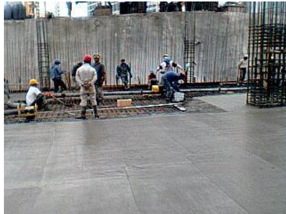
COLADO LOSA S2
