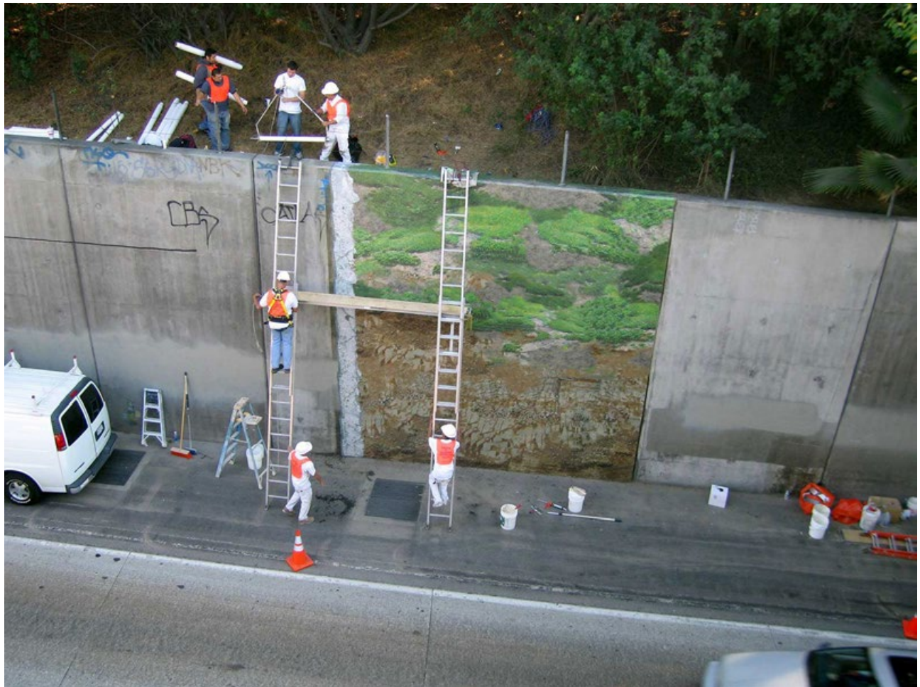
72. Freeway Wall Extractions , 2006
