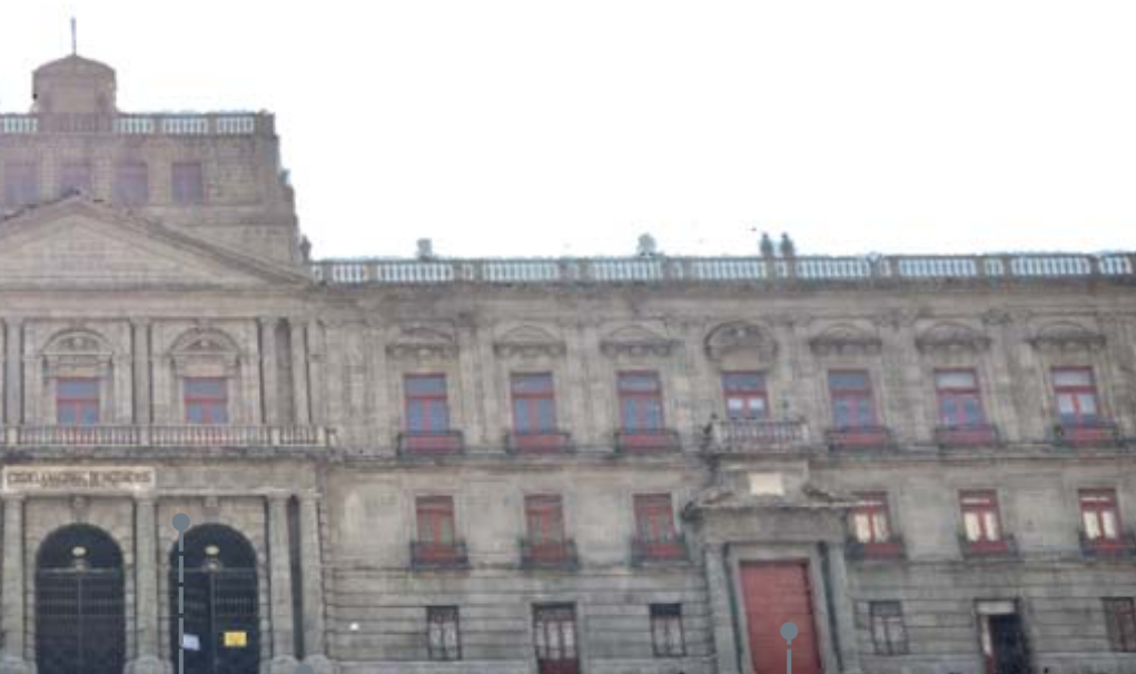
FACHADA PRINCIPAL Calle Tacuba
