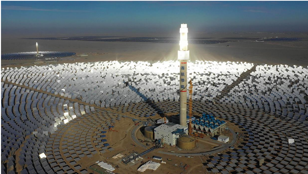
Figura 3. Central solar Shouhang Dunhuang 100 MW Phase II en Dunhuang, China.
