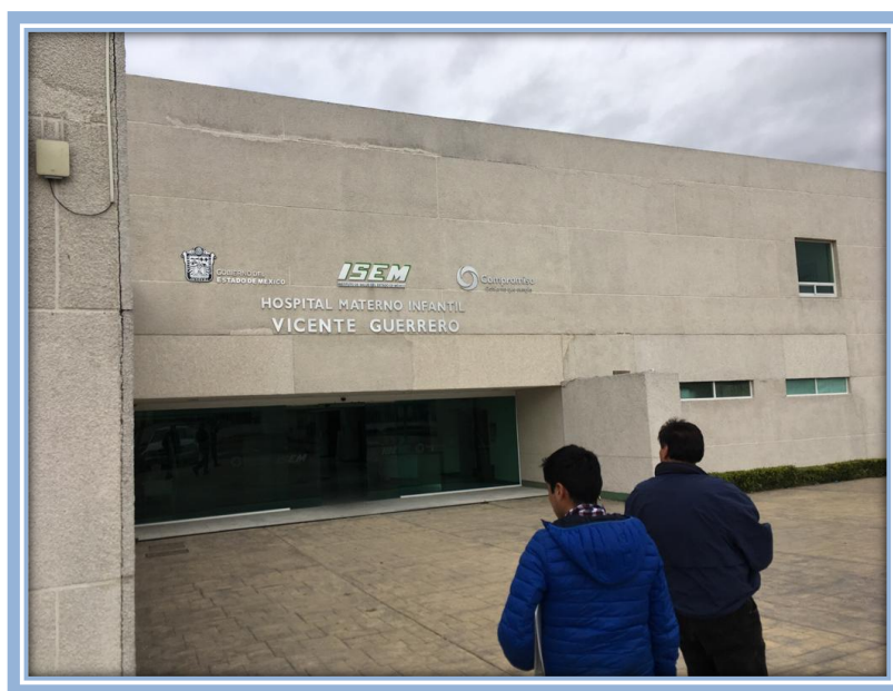
FIGURA 22 Fachada principal hospital materno infantil, Chimalhuacán
