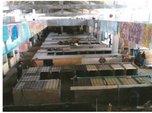
Fig. 8 Construction of bars for business tables
