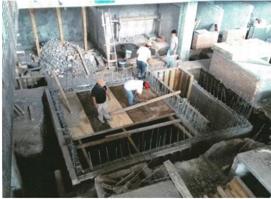
Fig. 7 Top slab formwork of the tank and the machine room
