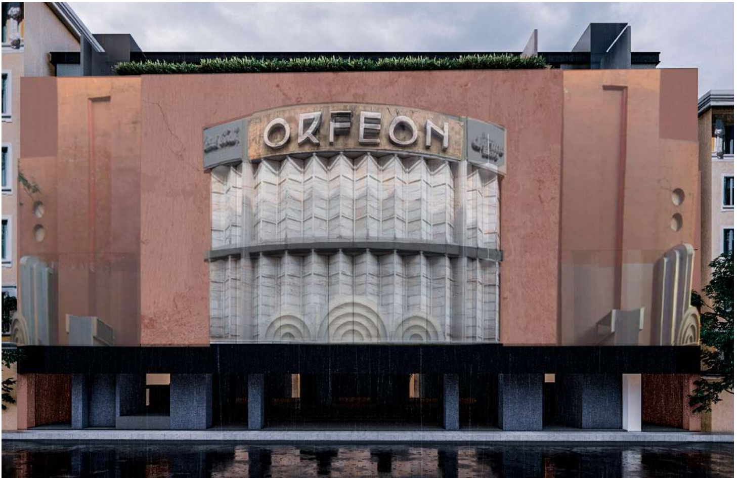
Fachada Principal | Vista frontal | Orfeon
