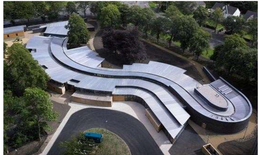
Foto 13: Escuela "Hazelwood" / "Hazelwood" School. (Archkids, 2011).
