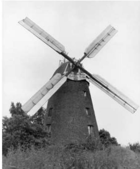
Figure 1.16. Windmill with subsequently added “Ventikanten” sails (photo Fröde)
