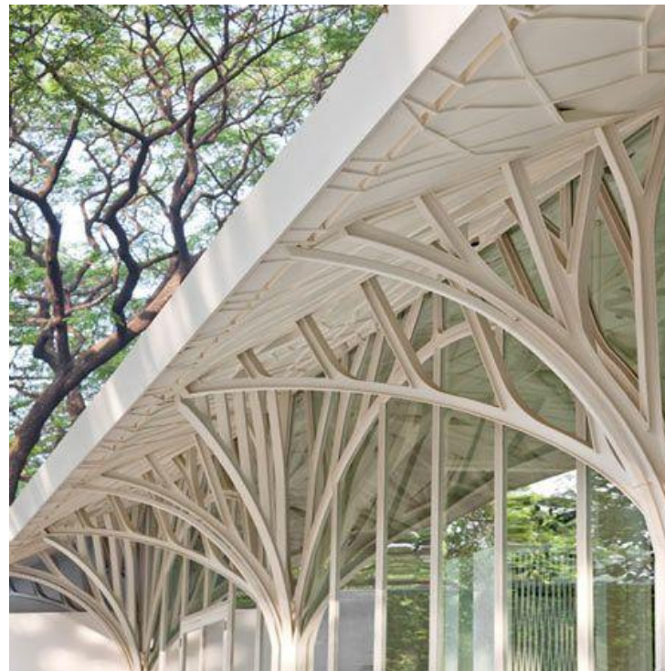
Columnas exteriores Restaurant "The Tote", Mumbai, India
