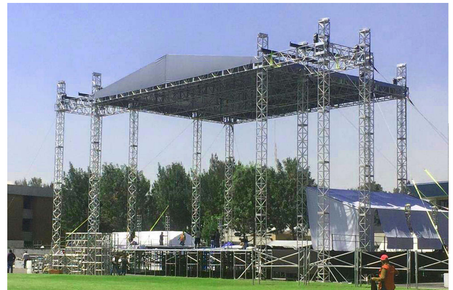
Escenario con sistema ground support. https://riggingplot.com/gs-4.html
