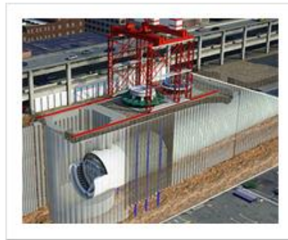
6. Lifting main components
