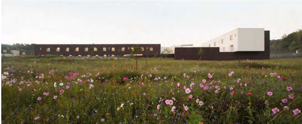
G. 63 92 camas, clínica de reposo, Dominique Coulon, ROMERO, D. (2015). Recuperado de: https://www.archdaily.mx/mx/782442/92-camas-clinica-de-reposo-dominique-coulon-and-associés?ad_source=myarchdaily&ad_medium=bookmark-show&ad_content=current-user
