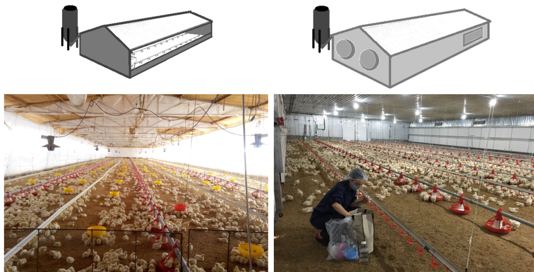
Figure 12. Two major types of housing systems in Mexican commercial farms: on the left, an open-sided type of barn; on the right, a controlled environment type of barn (personal photograph collection).
