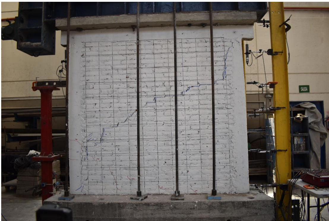
Figura 175. M-13 a \delta = 0.002 . Grieta pico: 4.0 mm, grieta residual: 2.0 mm.
