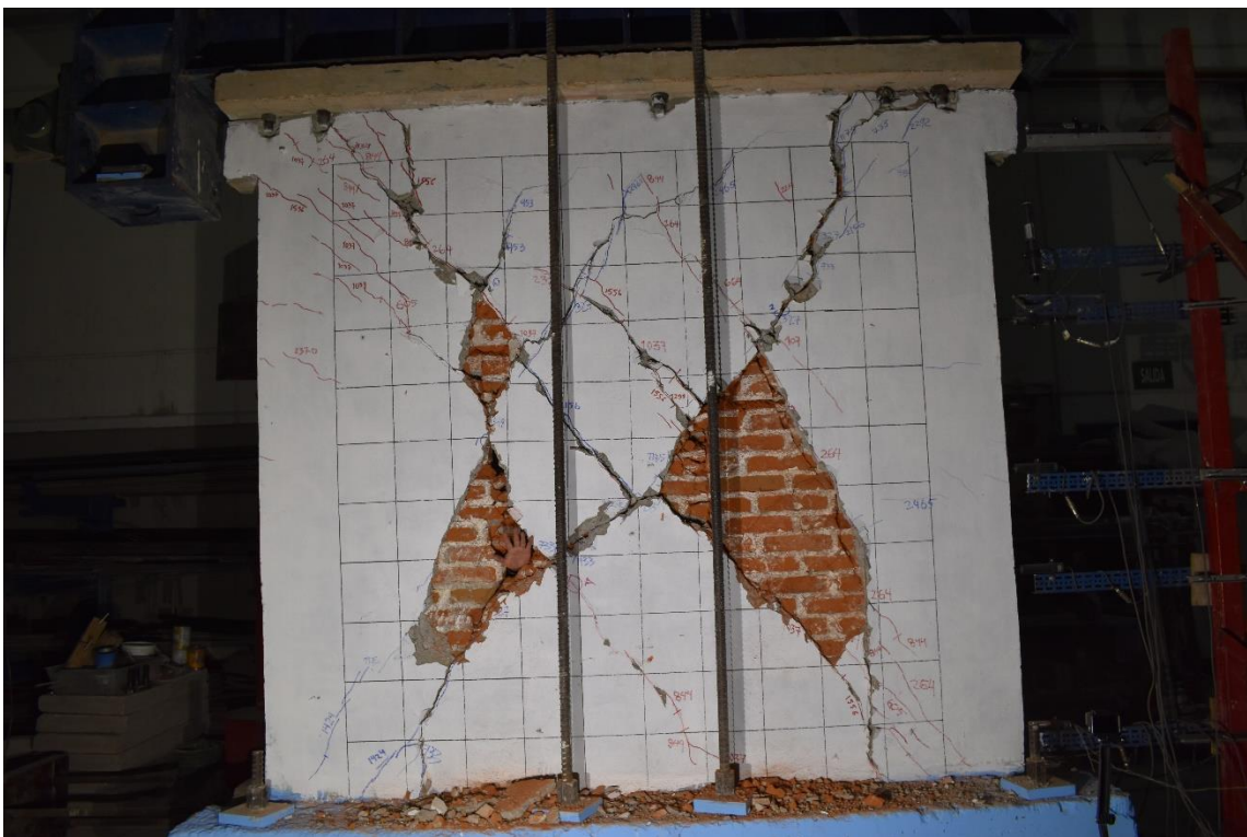
Figura 143. M-5R a \delta = 0.010 . Grieta pico 5.0 mm, grieta residual: 1.5 mm.
