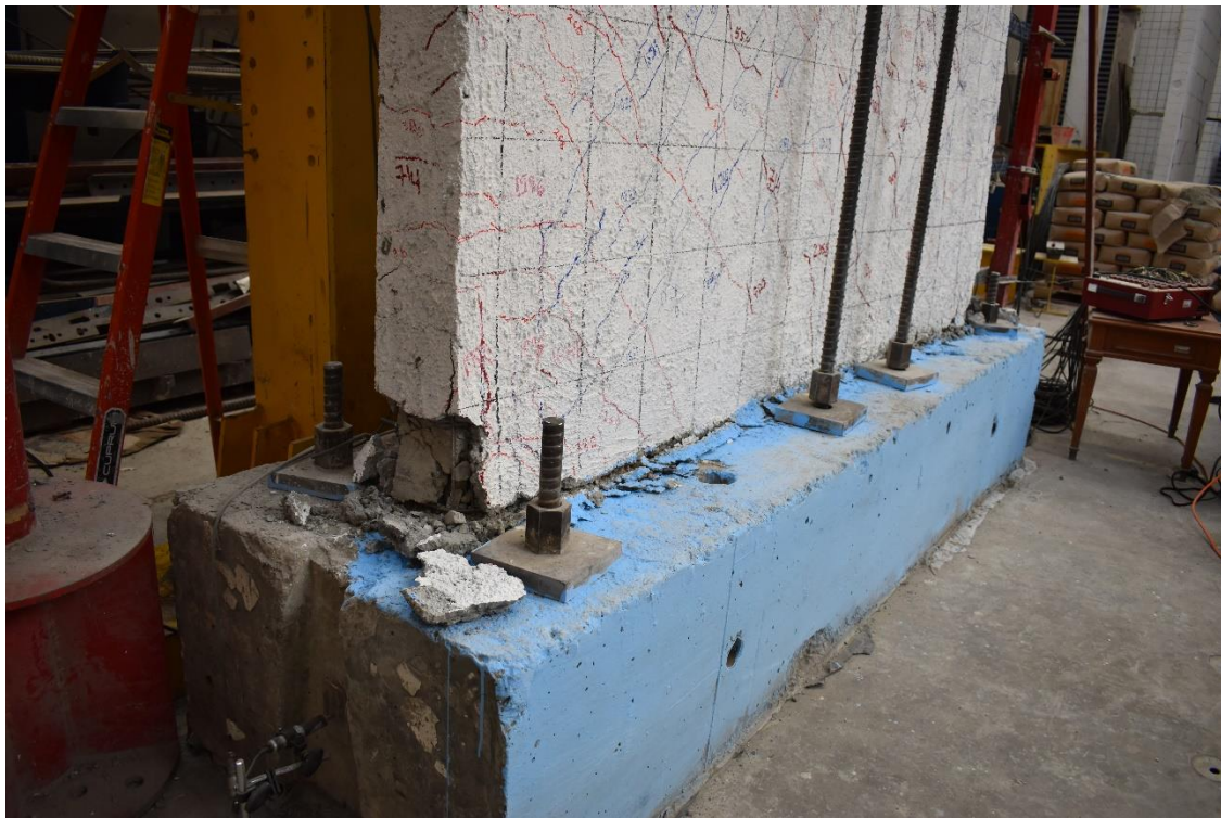
Figura 135. M-3R a \delta = 0.01 . Grieta pico: 0.2 mm, grieta residual: 0.1 mm.
