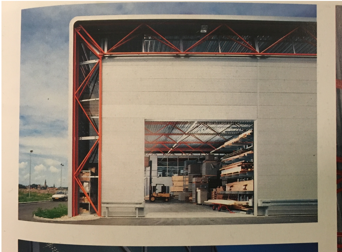
Imagen 9, Günel, Mahemet Halis. (2014). Tall buildings: structural systems and aerodynamic form / Mehmet Halis Günel and Hüseyin Emre Ilgin. London: Ed Routledge, Taylor & Francis Group
