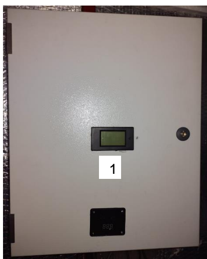
(a) Vista exterior
