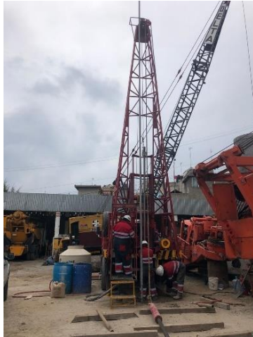
(a) Máquina perforadora Mobile Drill B621
