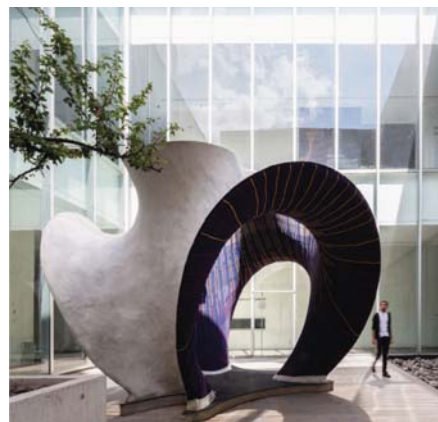
KnitCandela - A flexibly formed thin concrete shell at MUAC, Mexico City, 2018
