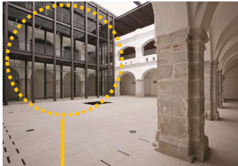
San Pablo Academic and Cultural Center / Taller de Arquitectura Mauricio Rocha + Gabriela Carrillo 14 Apr 2016. ArchDaily
