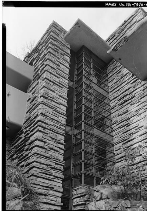
Fig. 21. Ventana vertical que conecta los tres niveles de la casa Library of Congress Prints and Photographs Division Washington, D.C., http://www.loc.gov/pictures/search/?q=fallingwater&co=hh
