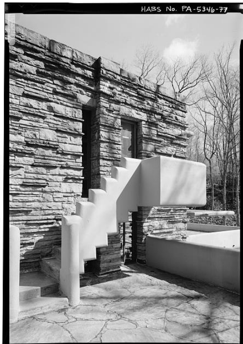
Fig. 24. Escalera exterior Library of Congress Prints and Photographs Division Washington, D.C., http://www.loc.gov/pictures/search/?q=fallingwater&co=hh
