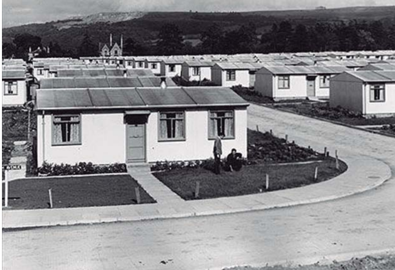
Figura, 210. A housing estate in 1940s England, where 173 aluminium prefab houses were built and occupied in just over 11 months. Recuperado de https://www.northcountrypublicradio.org/news/npr/94119708/www.cloudsplitter.org
