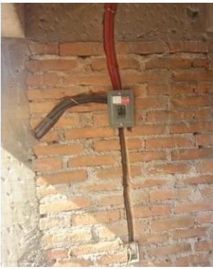
interruptor termomagnetico
