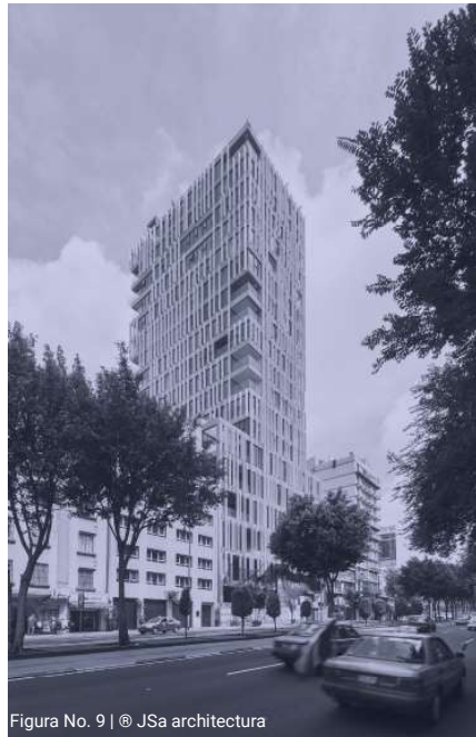
Figura No. 9 | © JSa arquitectura
