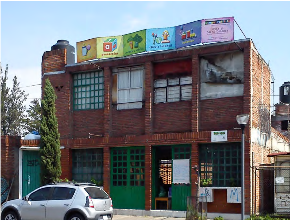
FIG_02 Fachada principal CECPP.
