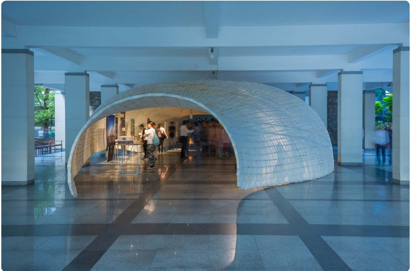
Fig. 13. 13.1, 13.2 y 13.3 - Pabellón en Vietnam Fuente: Santos, Sabrina. "Con 800 varas de bambú, A21studio contruye este pabellón en Vietnam" [A21studio Uses Bamboo and Poonah Paper to Build Cocoon Inspired Pavilion in Vietnam] 10 jul 2016. ArchDaily México. (Trad. Valencia, Nicolás) Recuperado de: https://www.archdaily.mx/mx/791092/a21studio-uses-bamboo-and-poonah-paper-to-build-cocoon-inspired-pavilion-in-vietnam
