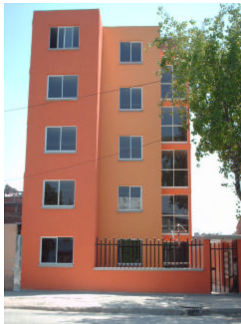
GUINEA NO. 64 FACHADA PRINCIPAL
