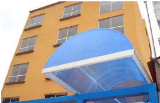
ERNESTO P. URUCHURTU NO. 86 FACHADA PRINCIPAL
