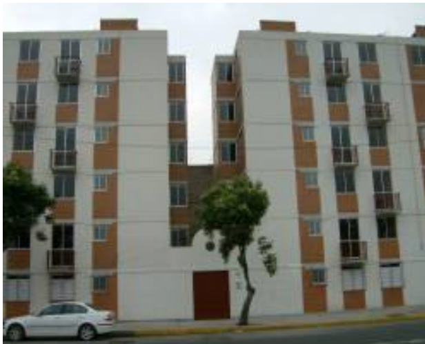
ERNESTO P. URUCHURTU NO. 86 FACHADA PRINCIPAL
