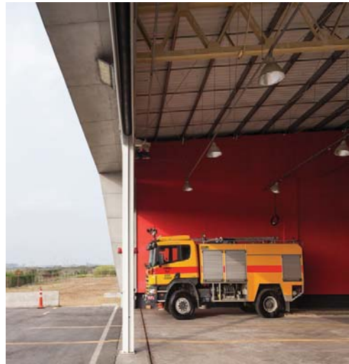
Ilustración 15. Guarulhos Airport Fire Department, São Paulo, Brazil https://images.adsttc.com/media/images/5b6c/6ebf/f197/cc4b/6200/001c/slideshow/20170814_mm18_gru_141.jpg?1533832881
