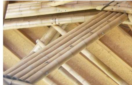
FOTO 1, VIGA COMPUESTA POR 5 BAMBUS
