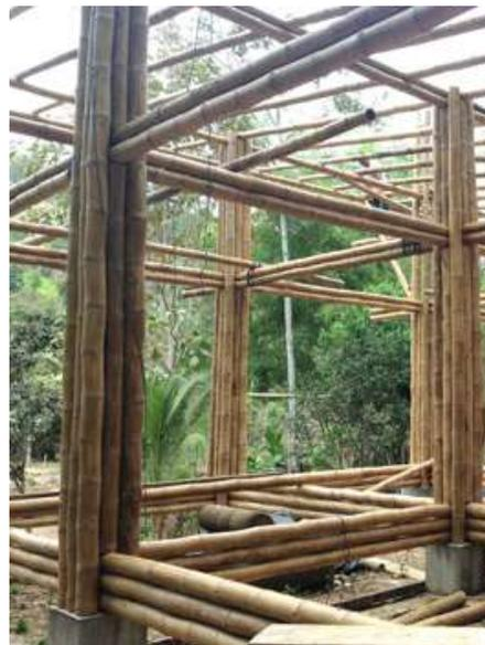
FOTO 7, COLUMNAS Y VIGAS COMPUESTAS
