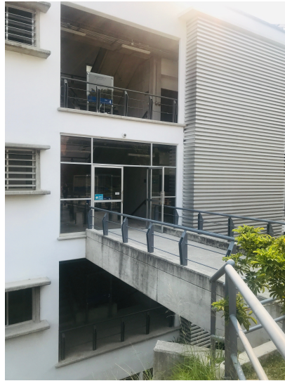
Figure 2.14: Photograph of the stairs zone in Building 3.1.
