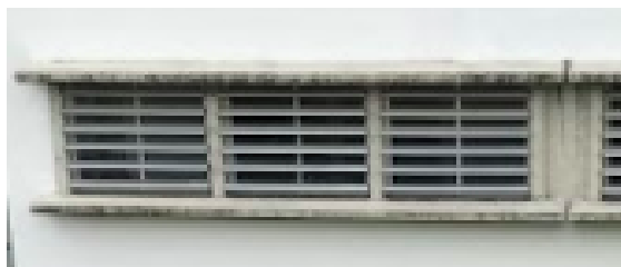
Figure 2.8: Photograph of Building 3.1 eaves.
