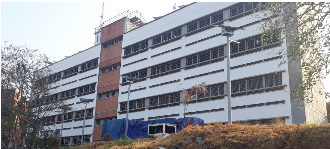
Figure 2.1: Real building view. Backside perspective.
