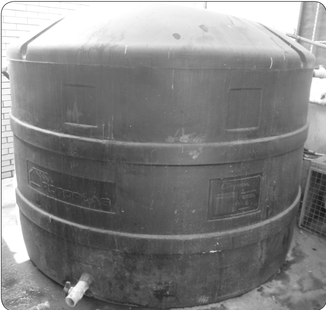
Figura 2.18 Reactor anaerobio R-II
