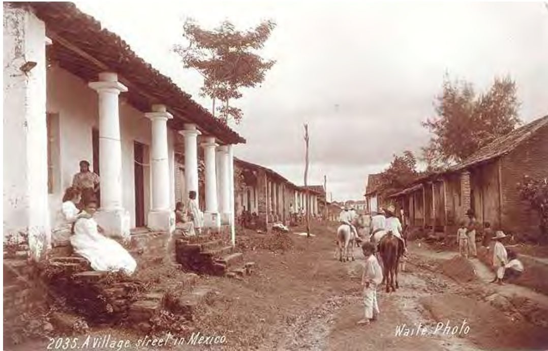
Figura 15 Viviendas construidas con tierra en México (B. Waite, A village street in Mexico, 2000).
