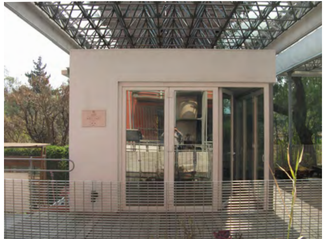
Fig. 85.1 Community: vista exterior norte
