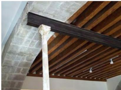
VIGA "T" Y COLUMNA METÁLICA
