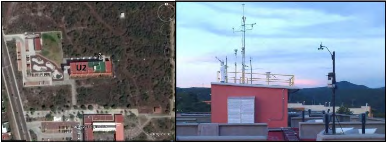
Figure 12: Location U 2 , aerial view (left) and view of the meteorological station on the rooftop (right).
