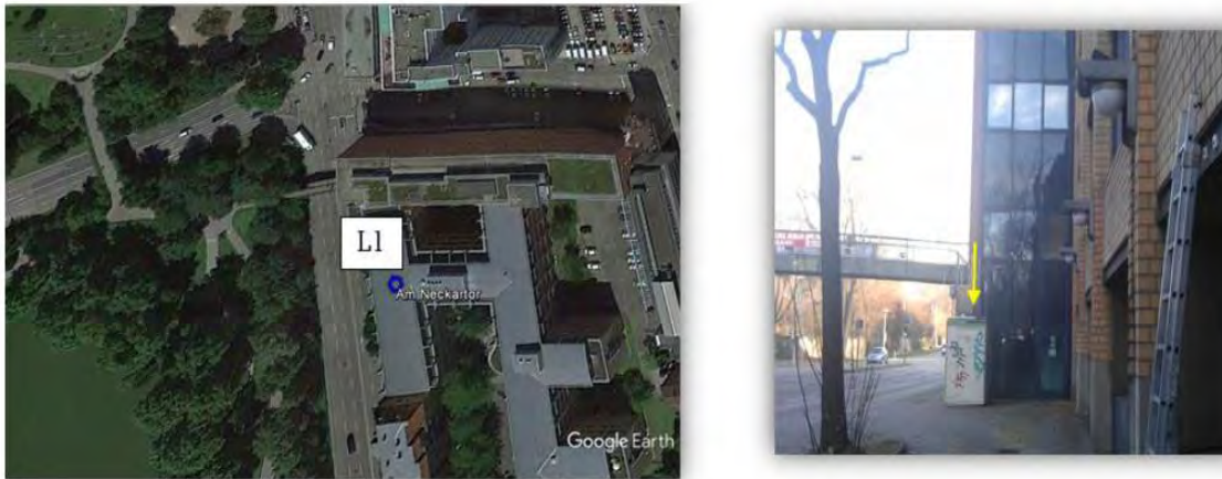
Figure 18: Aerial view of the location L_1 (left), close-up view to the location L_1 (right). The meteorological station is signaled with a yellow arrow. Magnets were attached to an iron surface 2 m above the ground, next to the ladder on the right figure.
