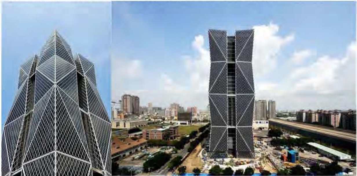
China Steel Corporation, Taiwan. Kris Yao, Arquitectos
