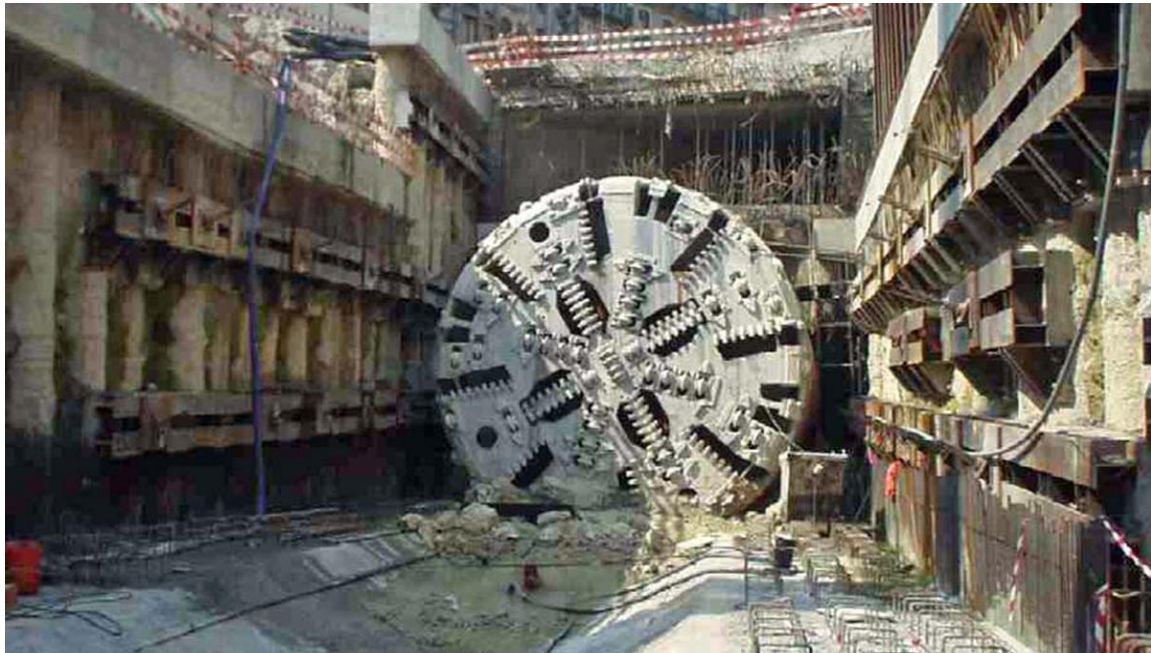
Fig. 1.6. Porto Light Metro Project 28
