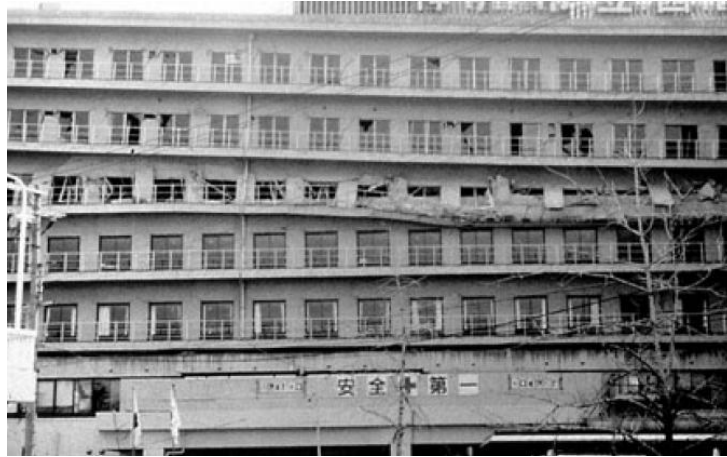
Figura 2.54 Hospital Municipal de Kobe
