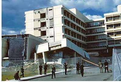
Figura 2.46 Hospital Olive View 1
