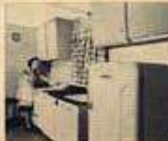
Kitchen includes all cabinets, cabinet top and combination dishwasher/dishwasher unit among the many features you get in the "delicious price" of the Lustron Home.
