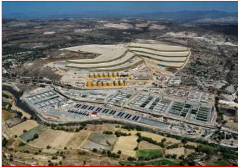
Figure 5.7. Atotonilco WWTP, Mexico (Taken from: CONAGUA, 2014)
