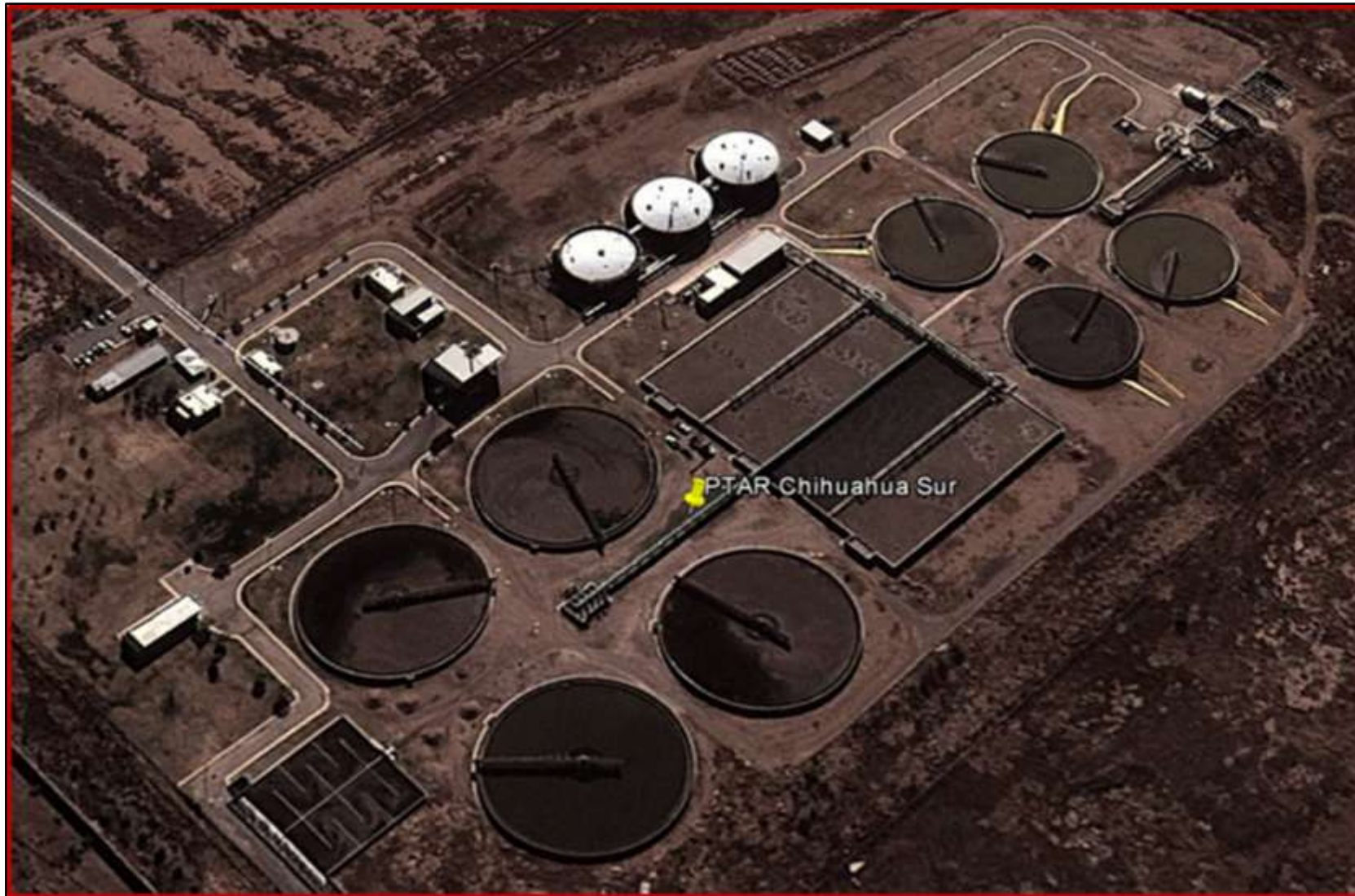
Figure 5. Aerial view of Chihuahua WWTP.
