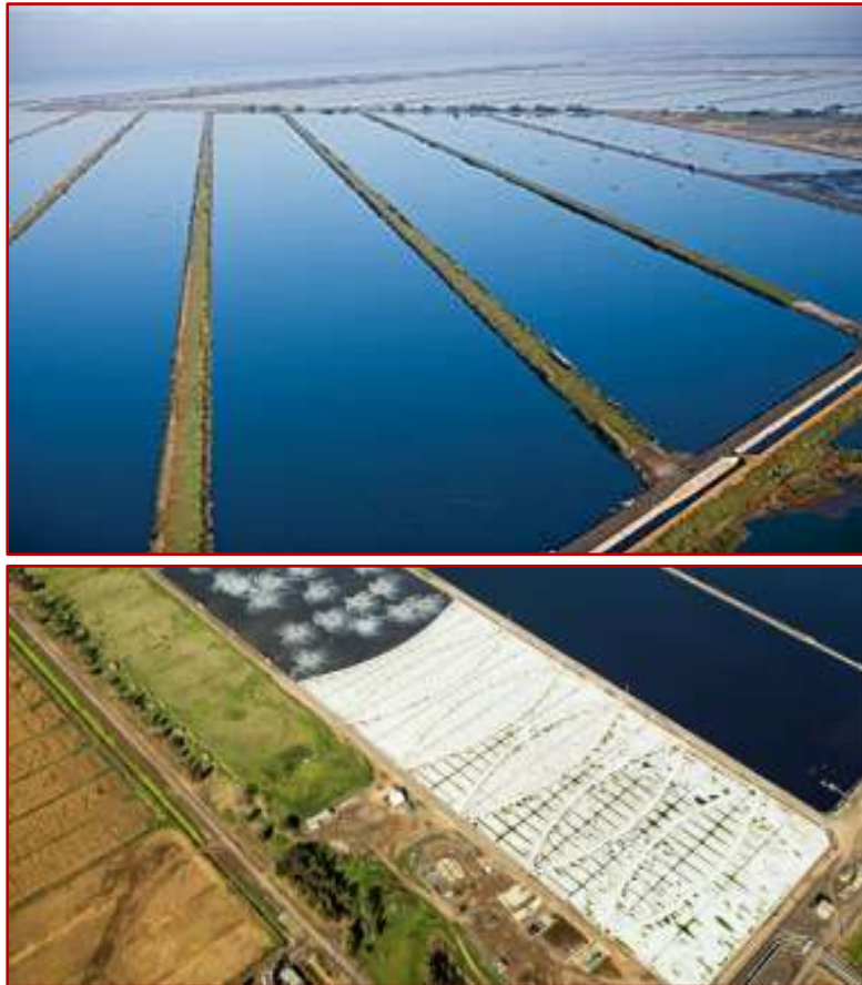
Figure 5.17. Melbourne WWTP, Australia with a view of the floating plastic cover (Taken from: Melbourne, 2007).
