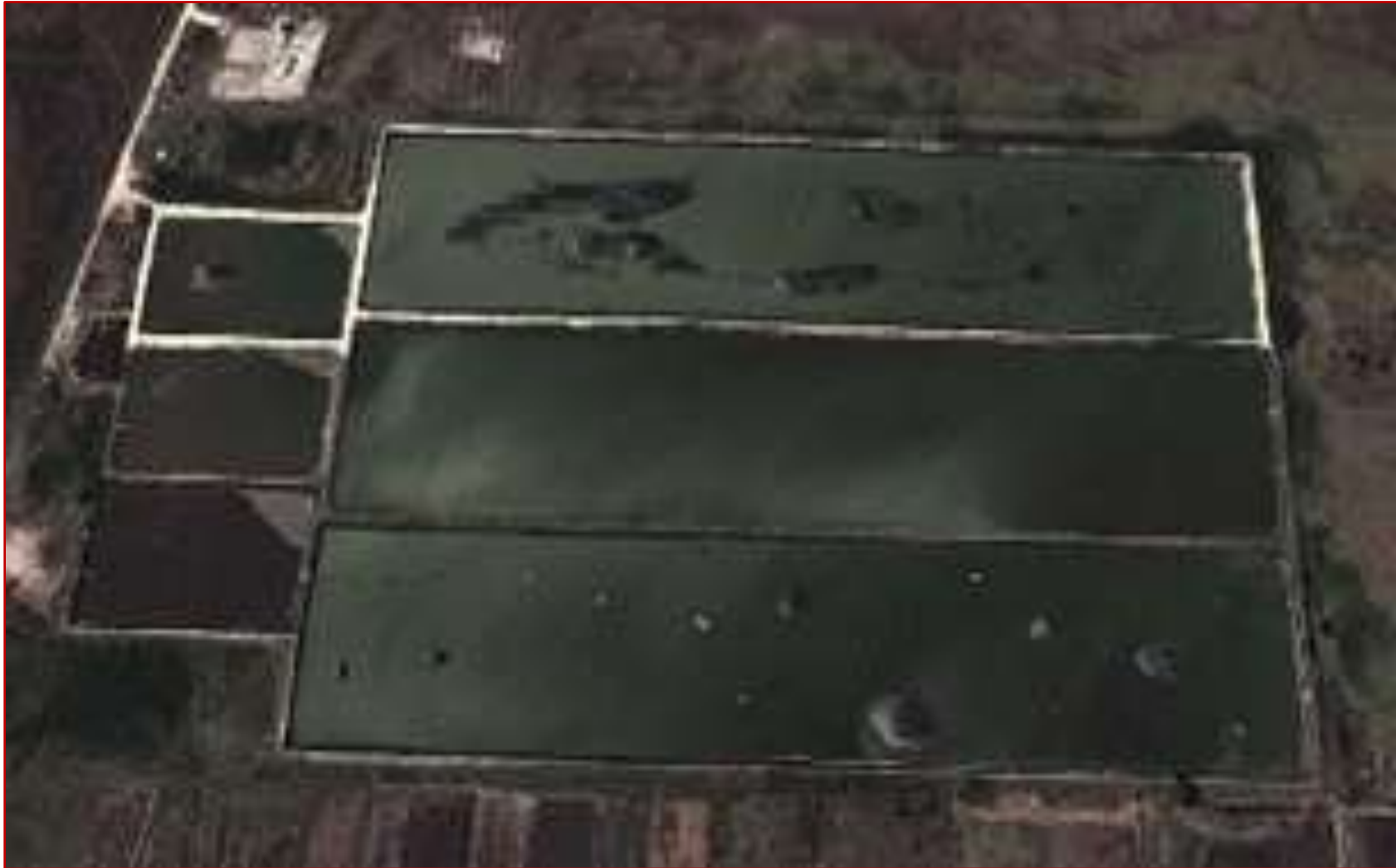
Figure 22. Aerial view of Comitán WWTP.
