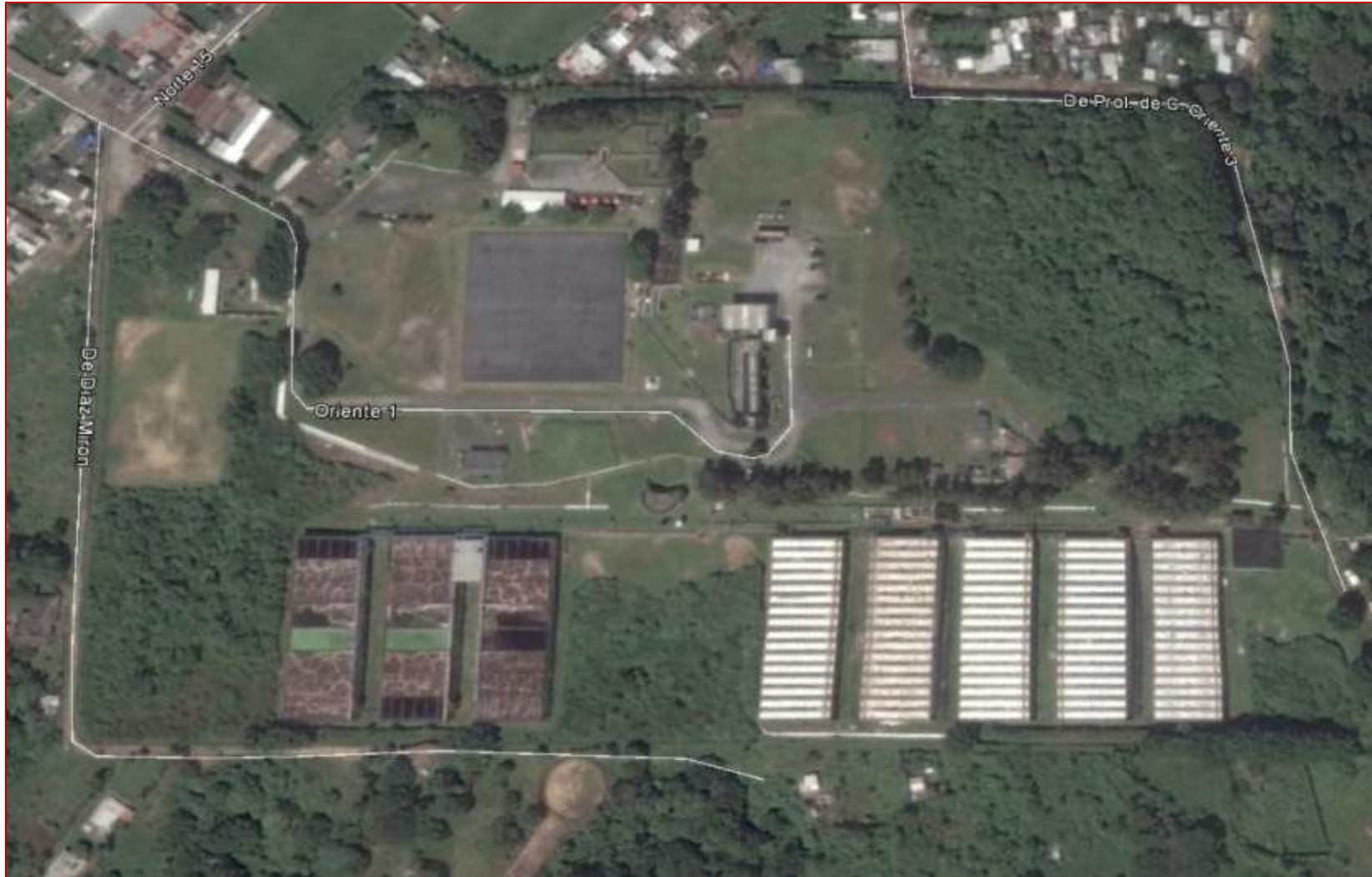
Figure 30. Aerial view of Veracruz WWTP.
