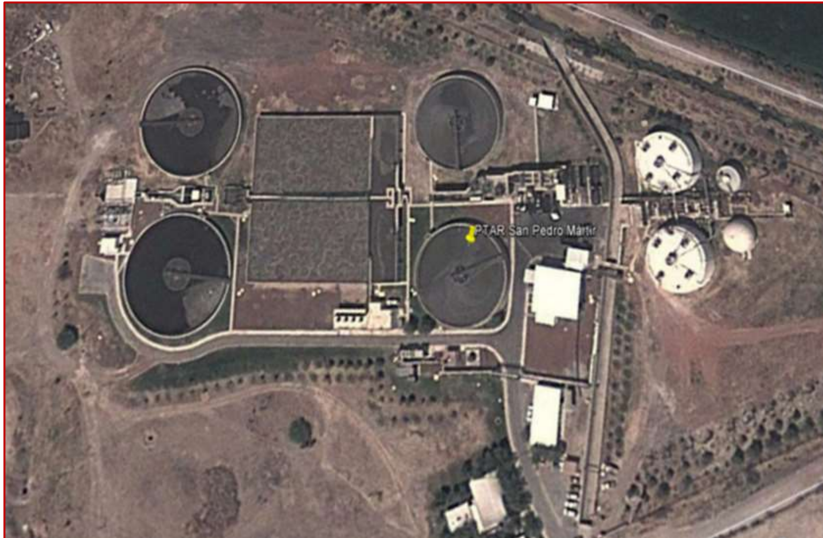
Figure 11. Aerial view of San Pedro Mártir WWTP.
