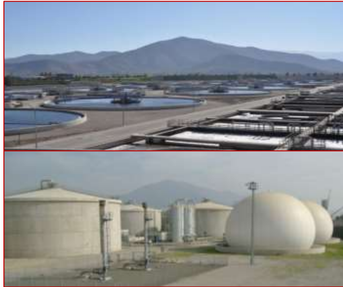
Figure 5.9. La Farfana WWTP, Chile (Taken from: GMI, 2012).
