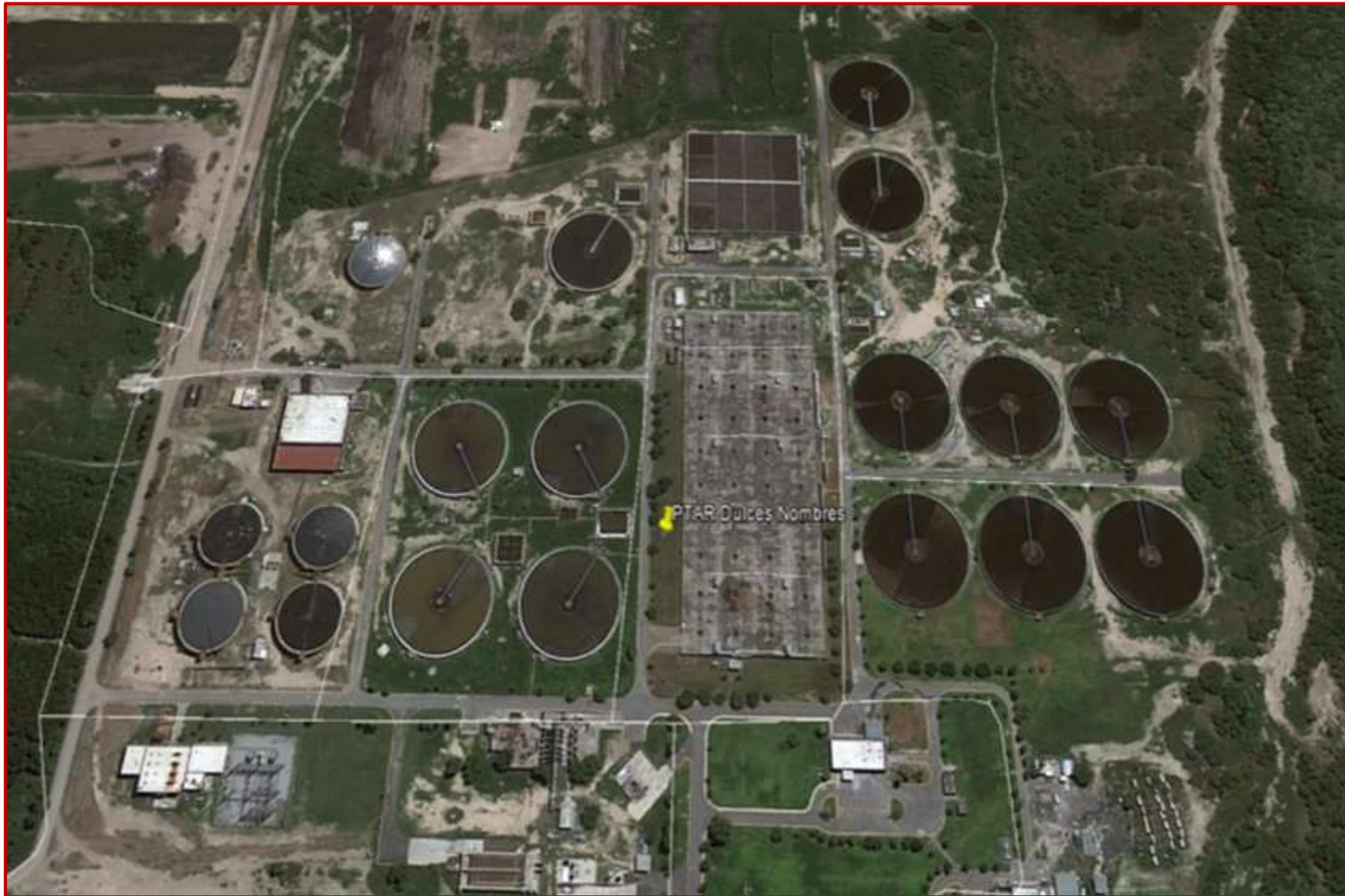
Figure 7. Aerial view of Dulces Nombres WWTP.
