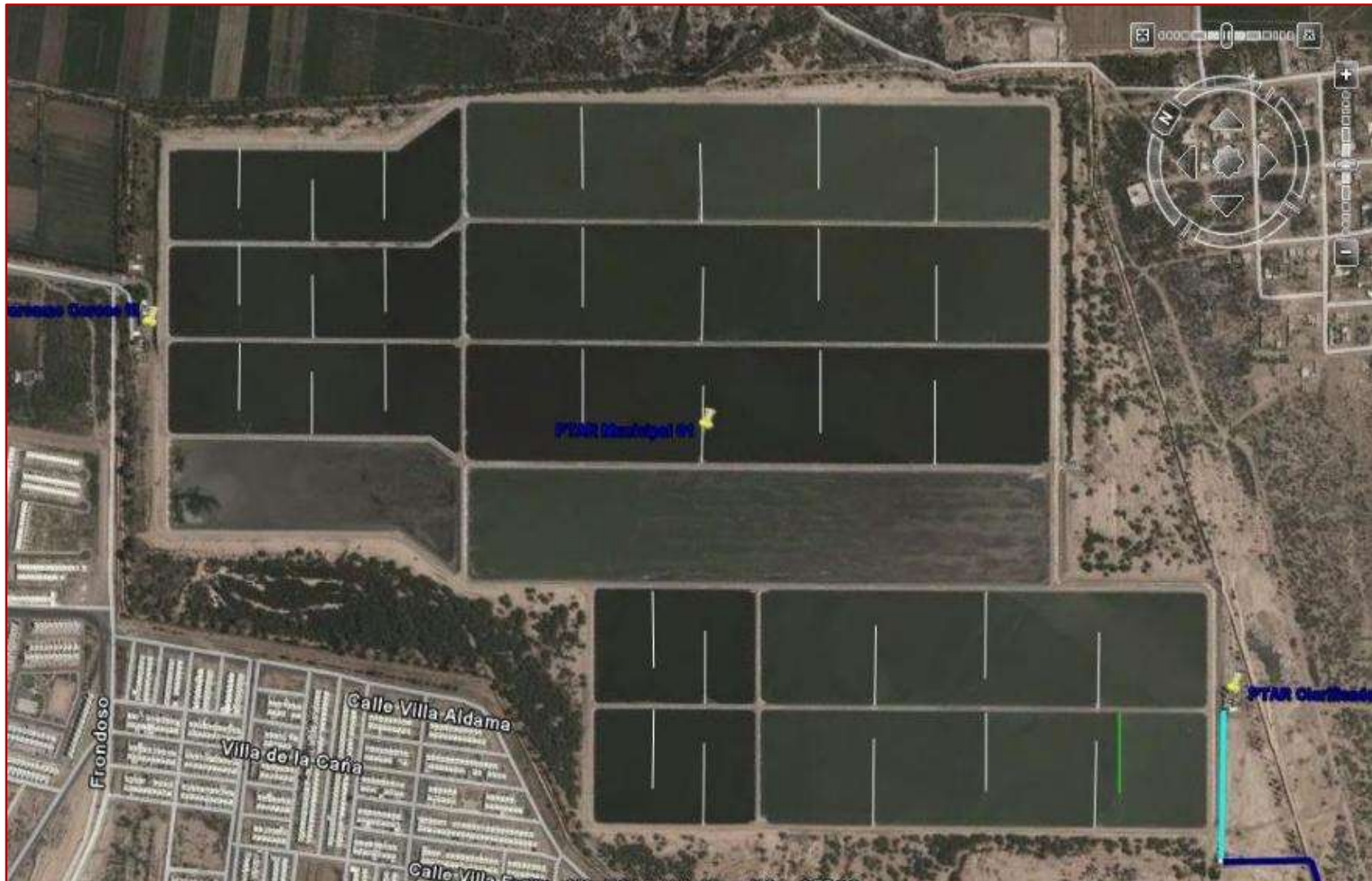
Figure 16. Aerial view of Torreon WWTP.
