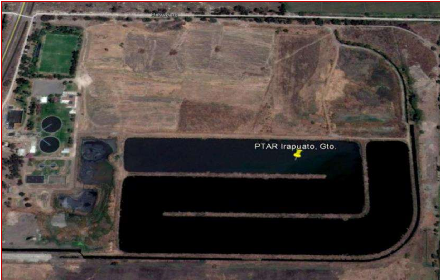
Figure 20. Aerial view of Irapuato WWTP.
