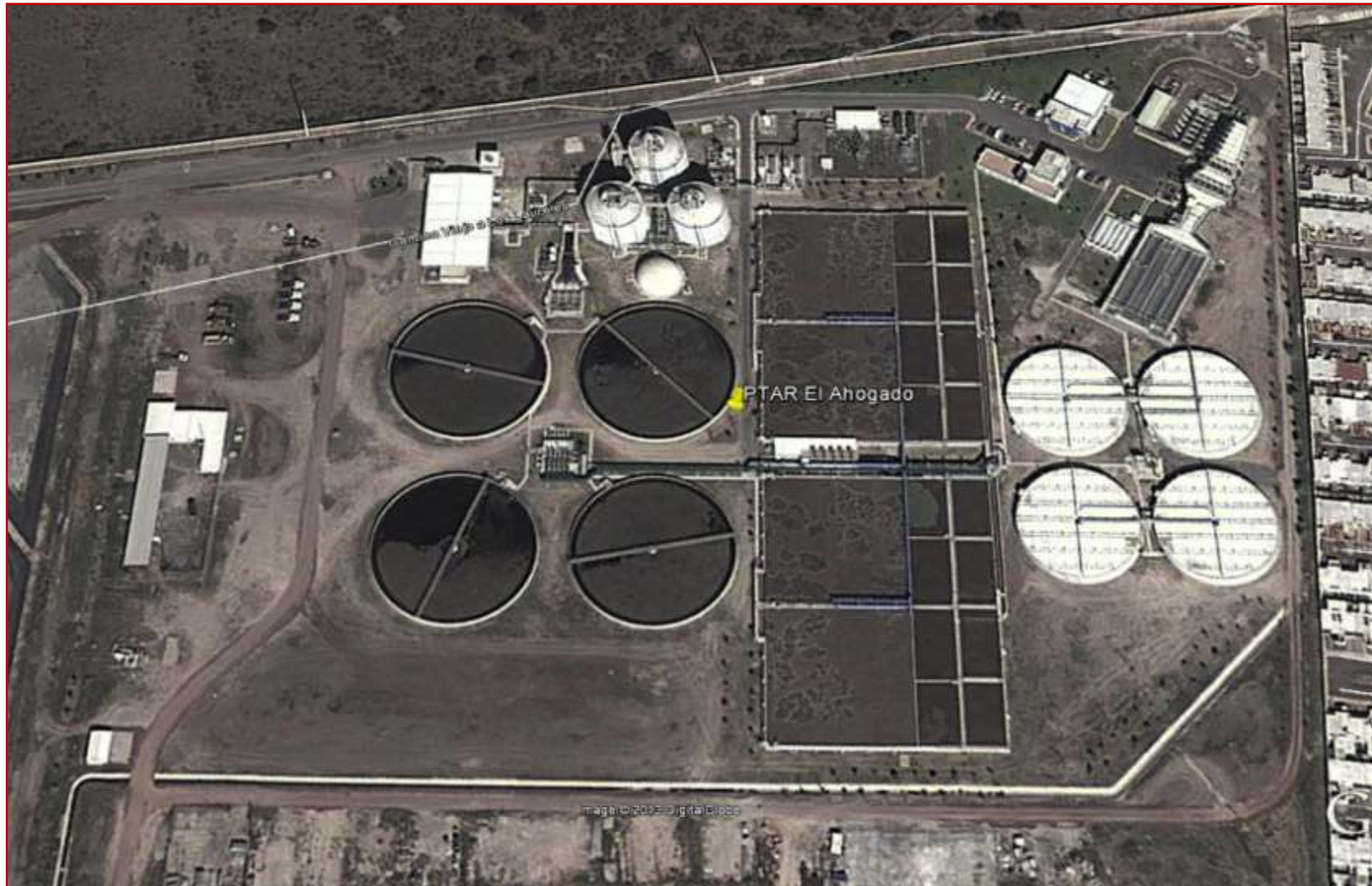
Figure 9. Aerial view of El Ahogado WWTP.
