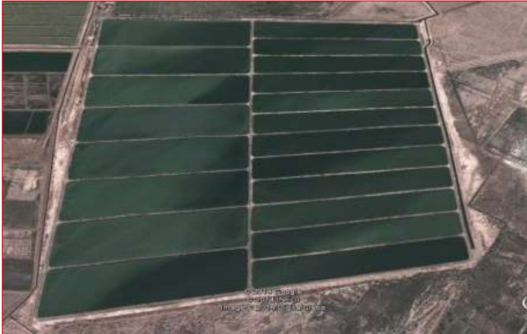
Figure 18. Aerial view of Los Mochis WWTP.
