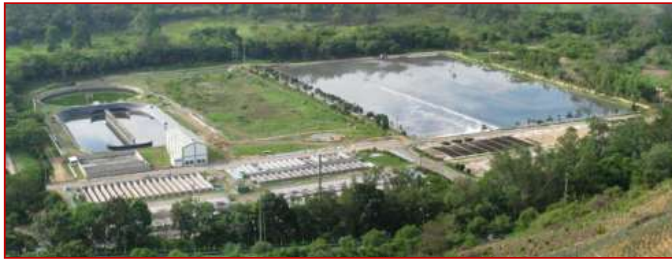
Figure 5.24. Rio Frio WWTP, Colombia (Taken from: EMPAS, 2013).
