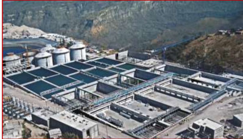
Figure 5.8. Agua Prieta WWTP, Mexico (Taken from: CEA JALISCO, 2013).
