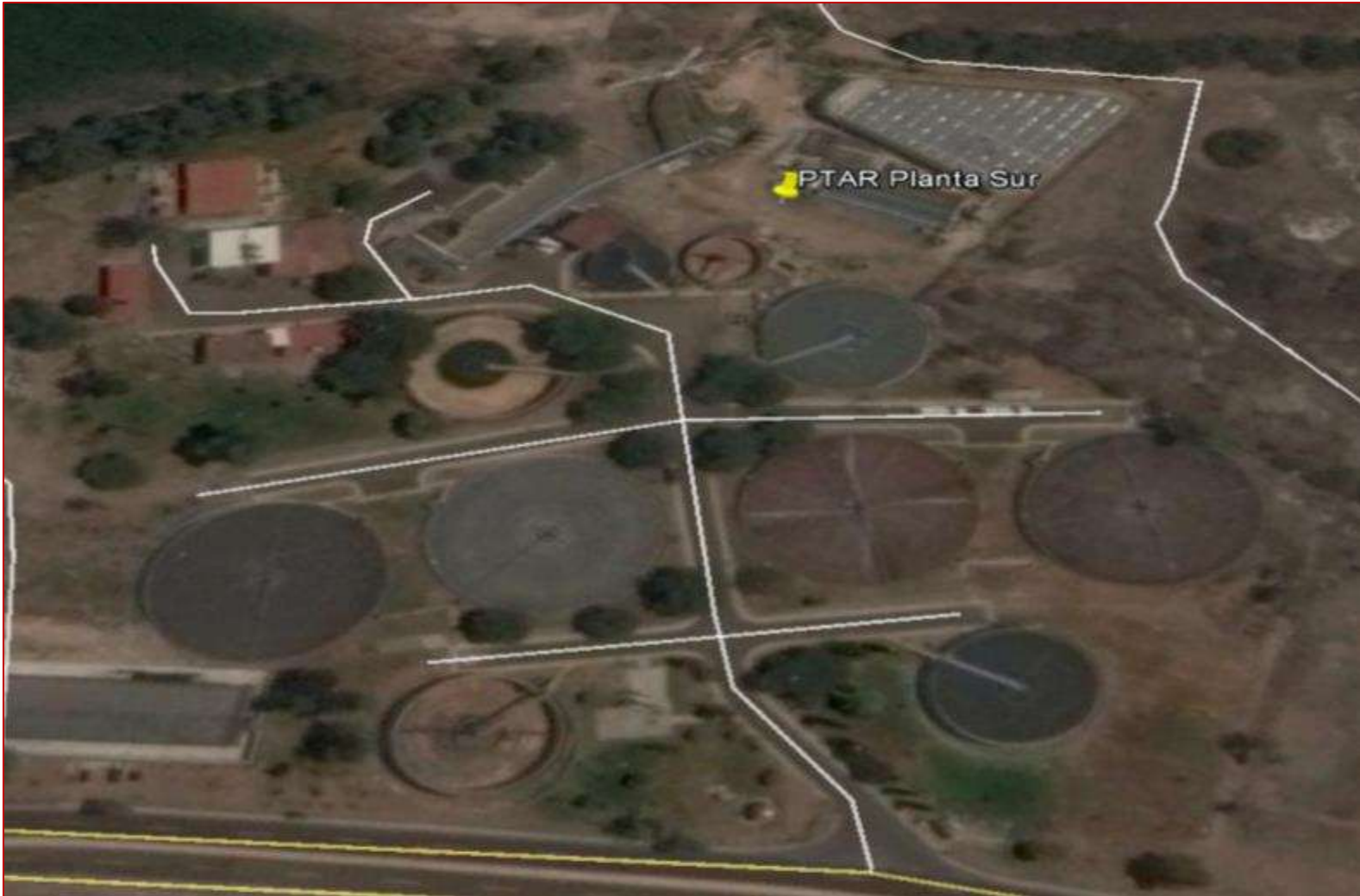
Figure 26. Aerial view of Queretaro Sur WWTP.
