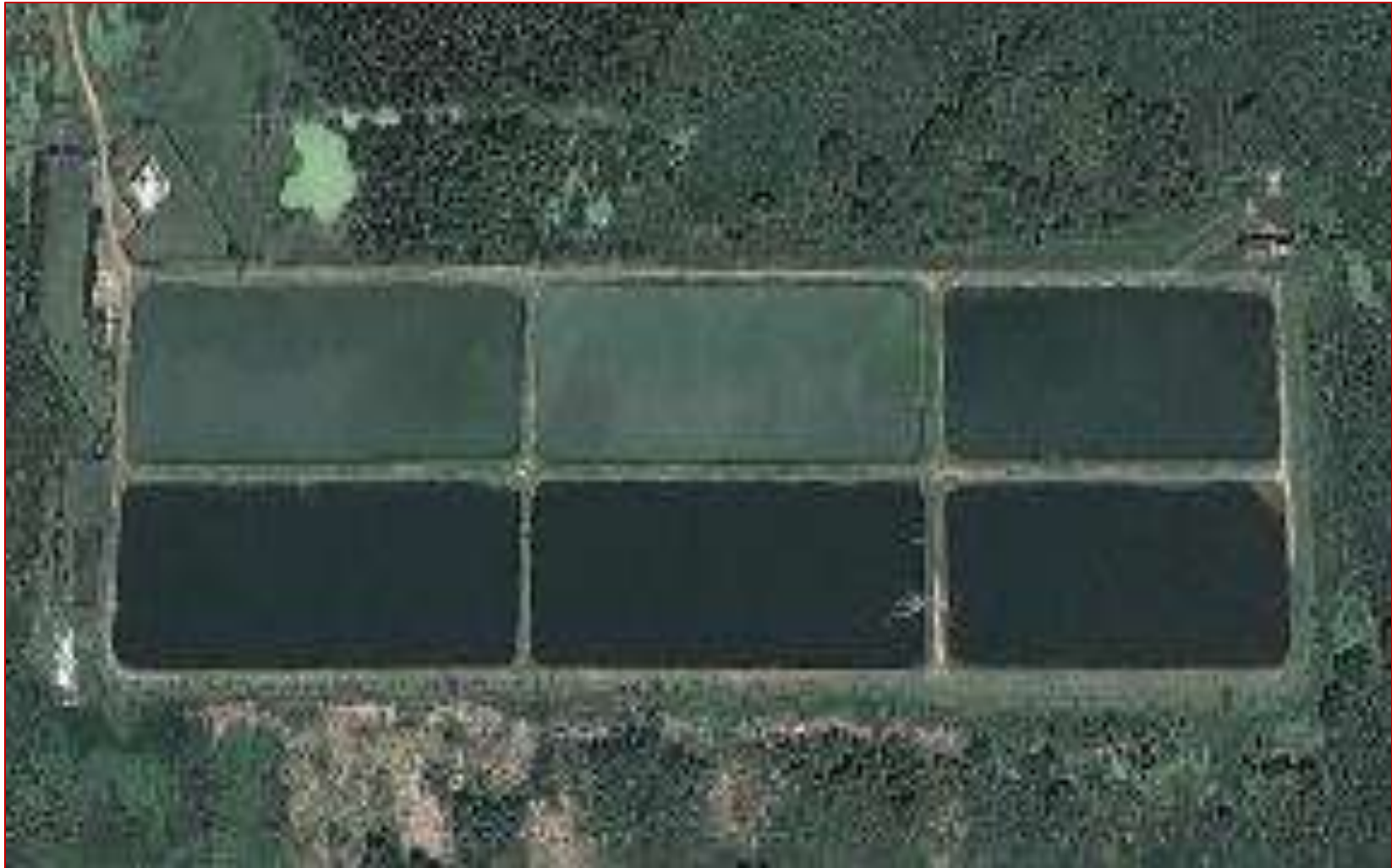
Figure 24. Aerial view of Veracruz WWTP.
