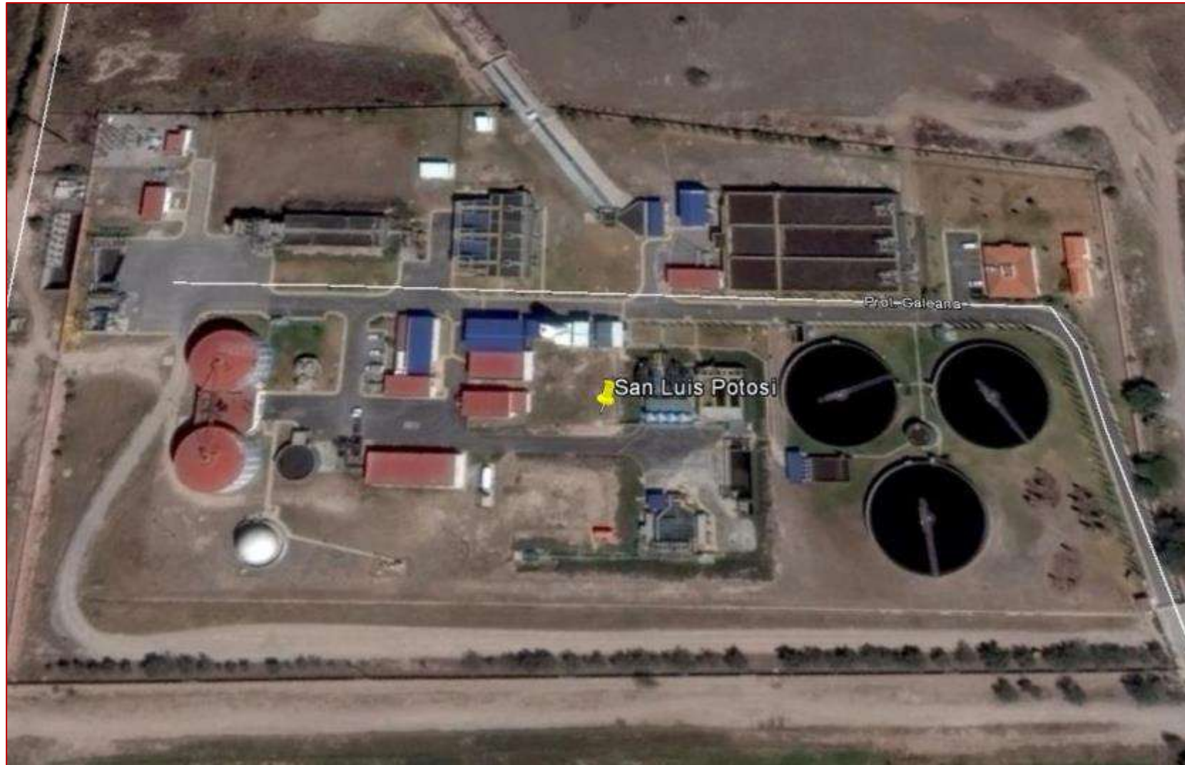
Figure 13. Aerial view of Tanque Tenorio WWTP.
