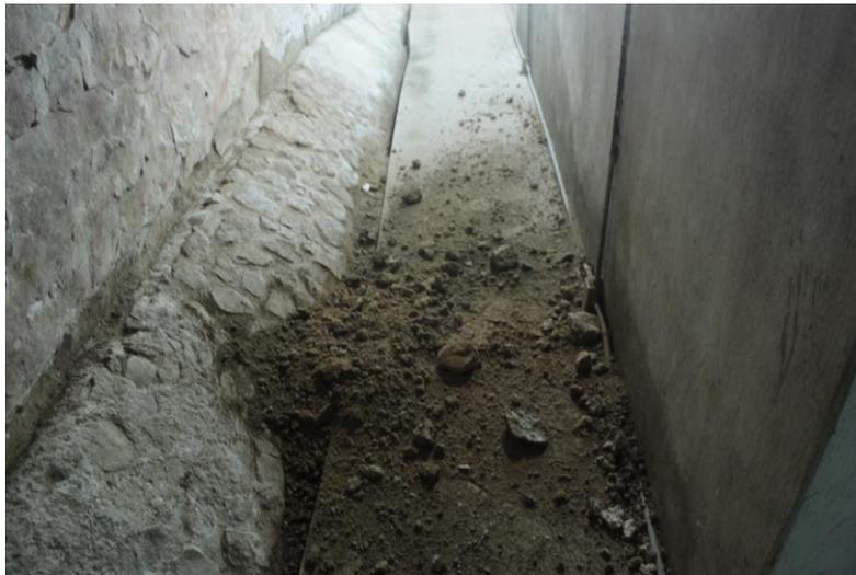
**Figure 3.** Detail of a collapsed earthen left upper wall of one of “Los Bebedores” mural that affects the stability and durability of the mural paintings.
