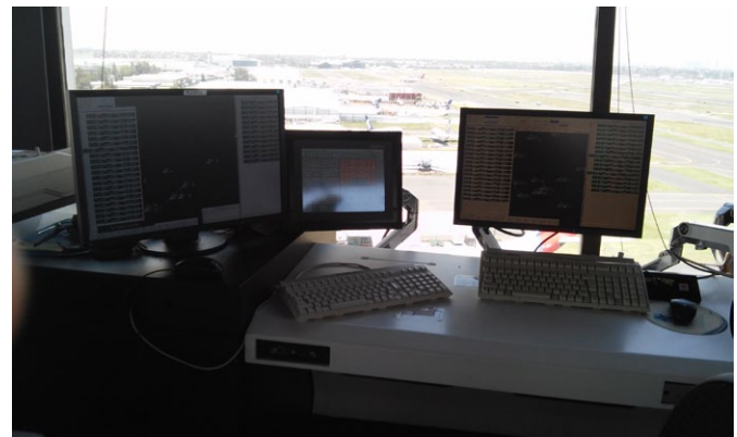
Figure 40: Unplanned installation of DRS.
